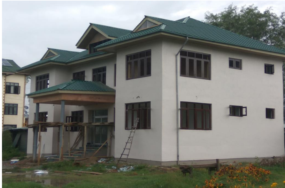
Fig.14: SSDI-JK building under construction at Bemina Office campus
